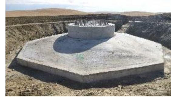
Each foundation requires approx. 400-600 m 3 of concrete
