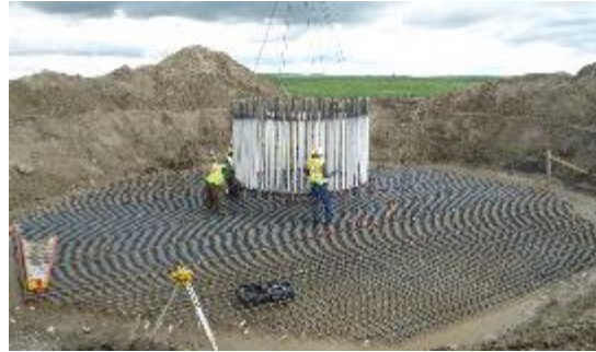
Reinforcing steel installation. Between 40-50 tons of rebar
