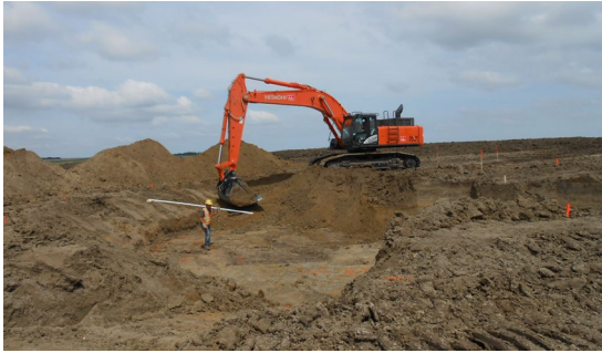
Foundation excavation. Diameter approx. 20 metres
